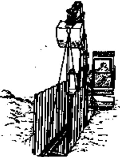
*A range of proprietary trench boxes and hydraulic wallings allow trench supports to be put in place without requiring people to enter the excavation.*
